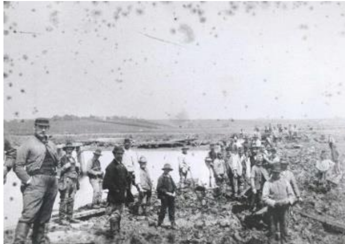
A photograph of workmen digging the Felixstowe dock basin. Credit: Hutchinsons Ports UK
